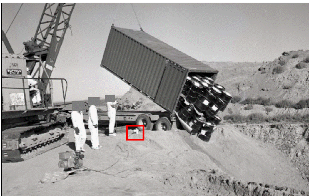
Figure B-5. 1969 photo of mass dumping of RFP waste drums with air sampling.
