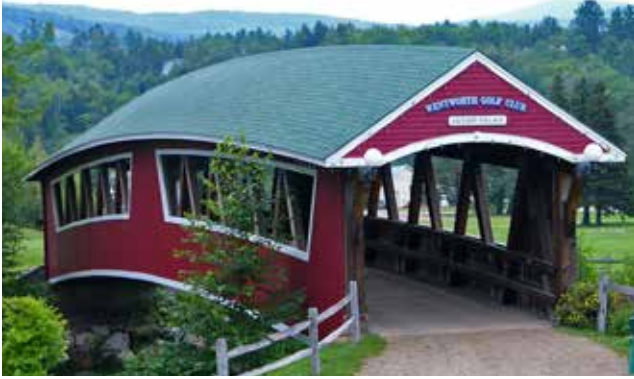
Photo Credit: NHDTTD/Anita Meissnitzer – Covered bridge at the Wentworth Golf Club in Jackson, NH
