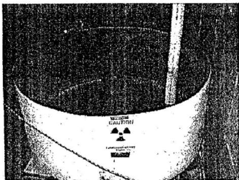
Photo #9 - Holding tank for wash down residue and water.
