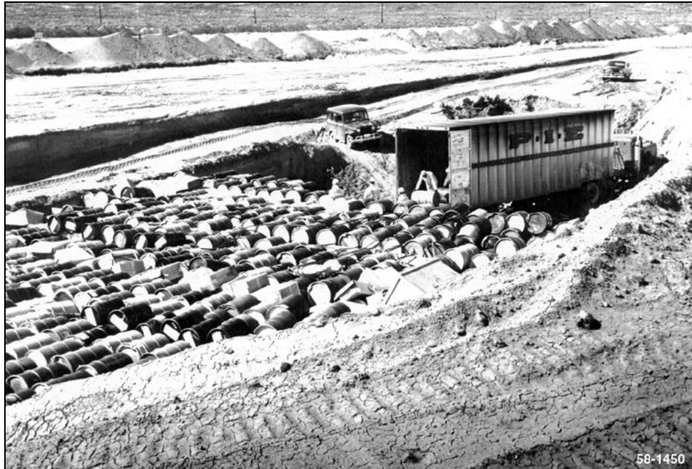
Figure 5-59: Emplacement of Rocky Flats Drums in a Burial Ground Pit in 1958
