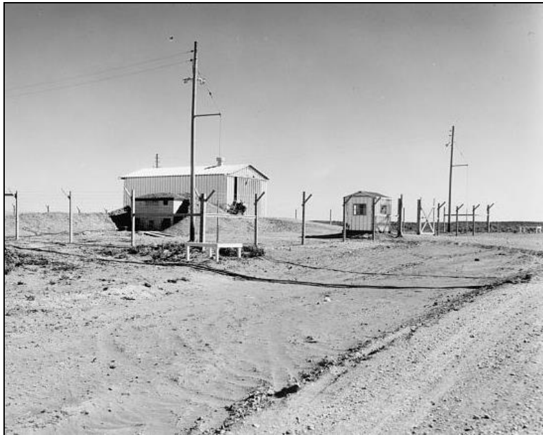
Figure 5-54: The SPERT-I Facility
