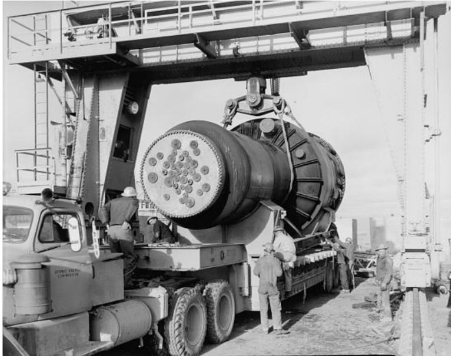
Figure 5-56: ETR Reactor Vessel Arriving at CFA Gantry Crane in 1956
