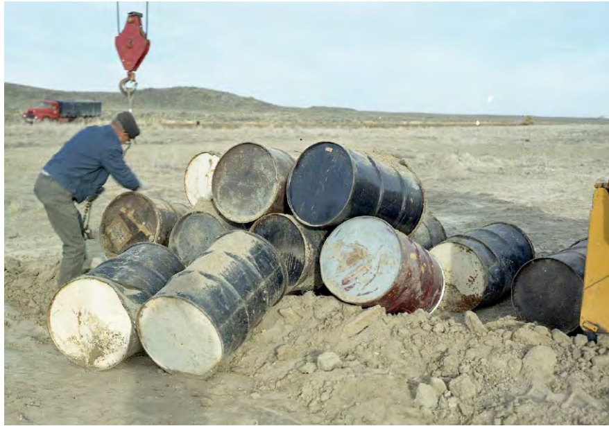
Figure 5-65: Burial Ground Health Physicist Assisting with Drum Retrieval from Pit 1
